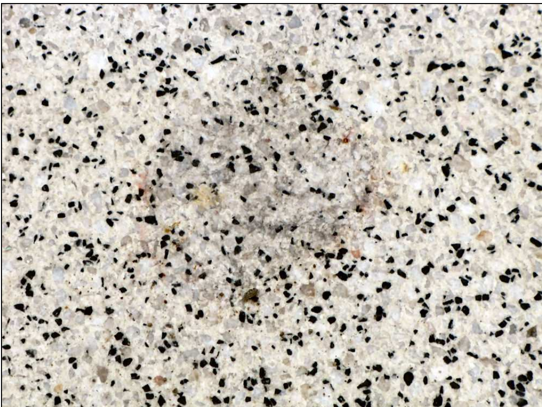
Figure 15 - Distinct damage to surface after 7 days in contact with paint stripper
