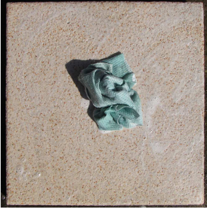
Figure 32 - Cleaning tyre marks using soapy water
