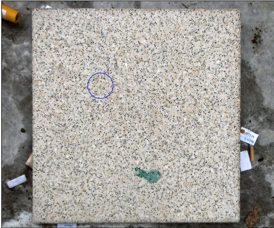
Figure 26 - Flag 3 after cleaning. Faint mustard stain is highlighted in blue circle
